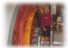
As a result, when Flanders built the new motors for the Logan mill, they made sure to include an Accumetrics Motor Monitor to constantly monitor the temperature of the armature. By continuously monitoring the internal temperature of the motors, the motors can run at a safe but full rating. Additionally, the mill operators can shut down the mill before a rise in temperature causes damage that would require an expensive and time-consuming rebuild.
