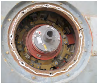
Figure 3 – Installations of EFREM on GE 7A6 units
