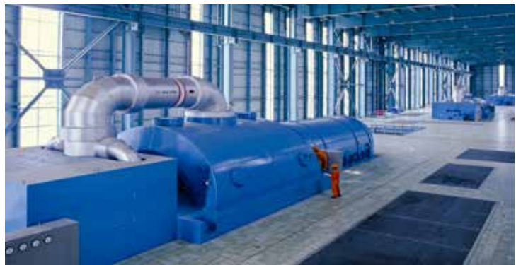
In the picture above, the EFREM transmitter is mounted to the end of the generator shaft, a flat plate is used to mount the stationary pickup coil.
